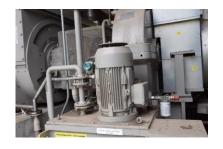
SEIMENS MANUFACTURE GENERATING 2.5Kw, year 2016 Model SST-060,1500 rpm, AFA6 G6B Exhaust steam min 1.5 norm, 2.5 max 4.1 bar Number 4.3666.045 1635 trip speed Type SST-060 AFA 66B
